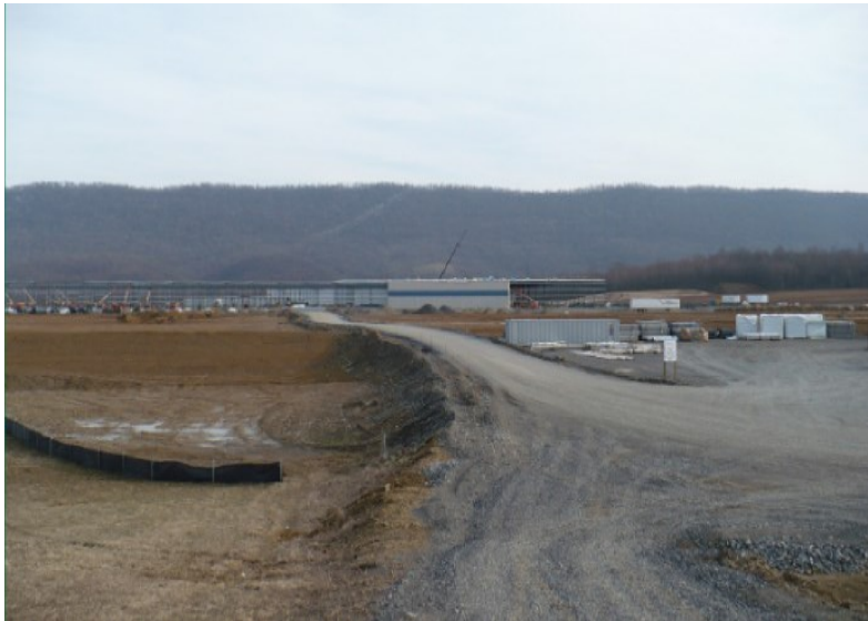
December 2007—Facility Being Erected
